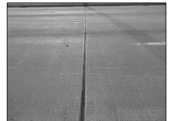
STRIP SEAL JOINT AT BENT LC7
